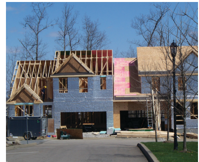
New housing under construction.
