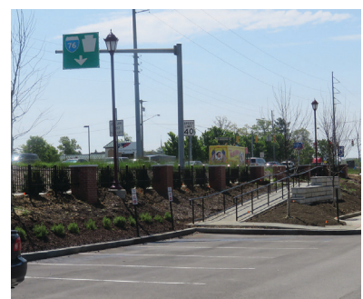
Streetscape enhancements outside of Jason's Deli at the Cranberry Mall.
