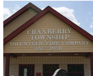
Two Volunteer Fire Stations service Cranberry Township.
