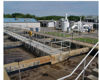
Capital improvements include Brush Creek Treatment Plant upgrades.
