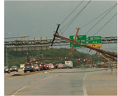
Strong winds downed power lines along Route 228 in 2014.
