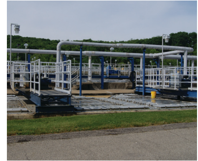
Brush Creek Water Pollution Control Facility
