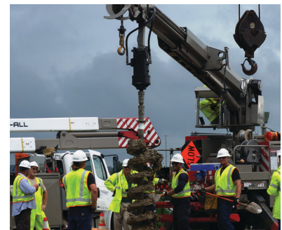
Teams worked around the clock to re-open the Route 228 roadway.
