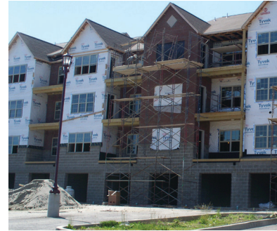
Multi-family units under construction.
