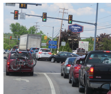
Turning lanes added to busy intersection on Freedom Road.
